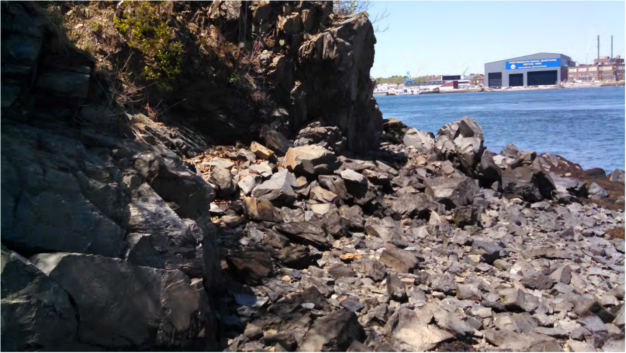
Photo 8 Proposed revetment 1, view north
